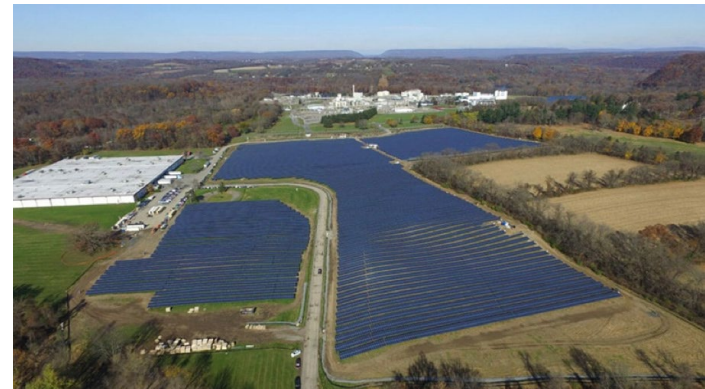
66-acre solar field in Belvidere, New Jersey, USA.
