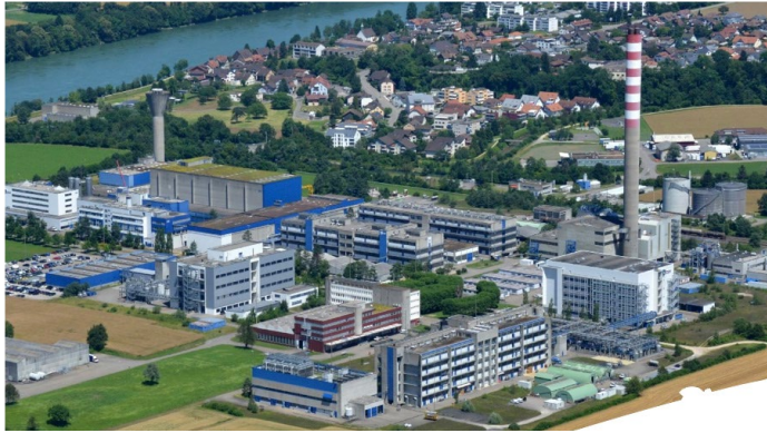
Woodchip-fired power plant in Sisseln, Switzerland.
